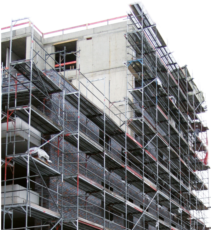
Pipe scaffold system
